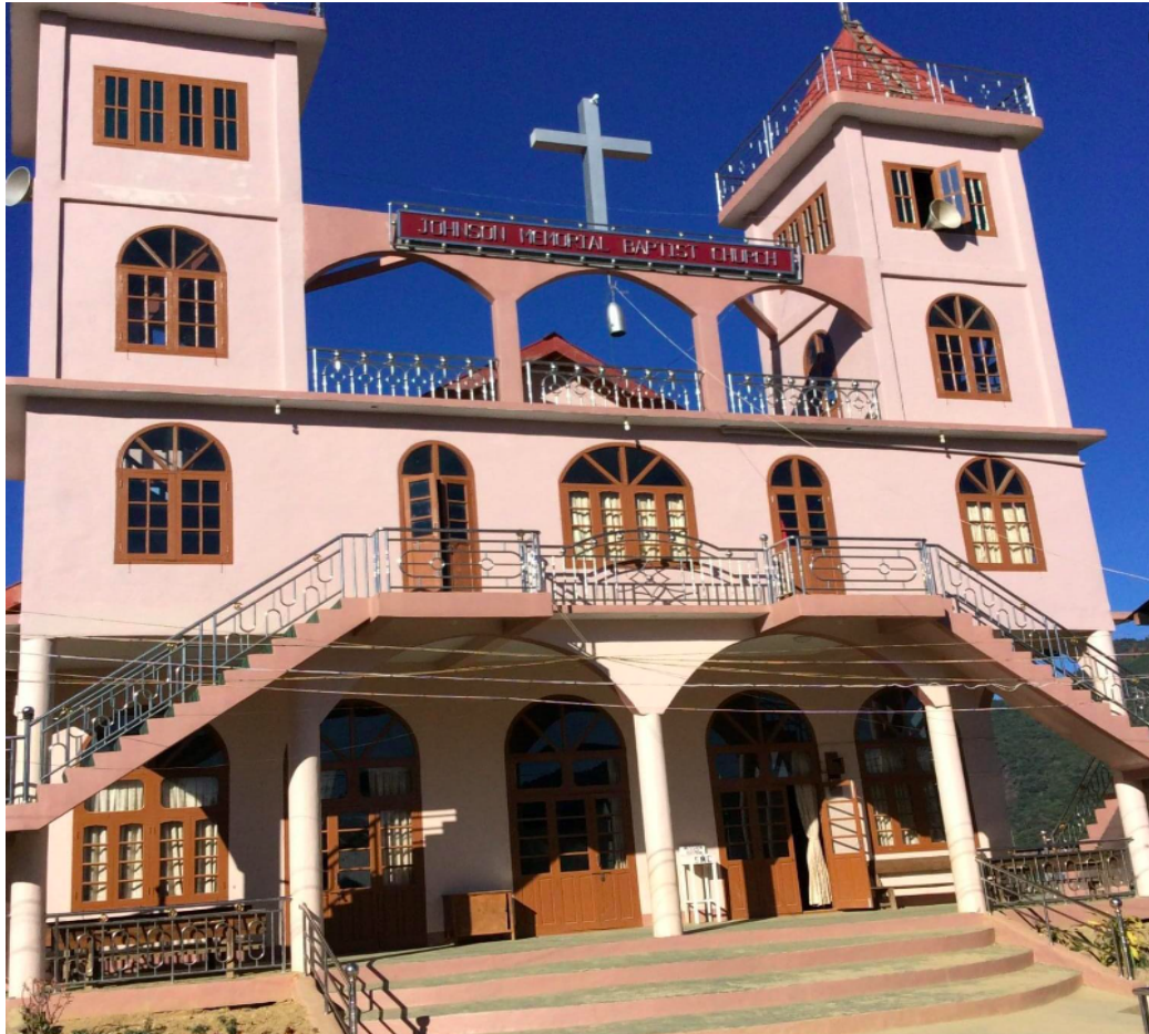
Photograph 11. The Johnson Memorial Baptist Church before it was completely burned down by the Myanmar military.
